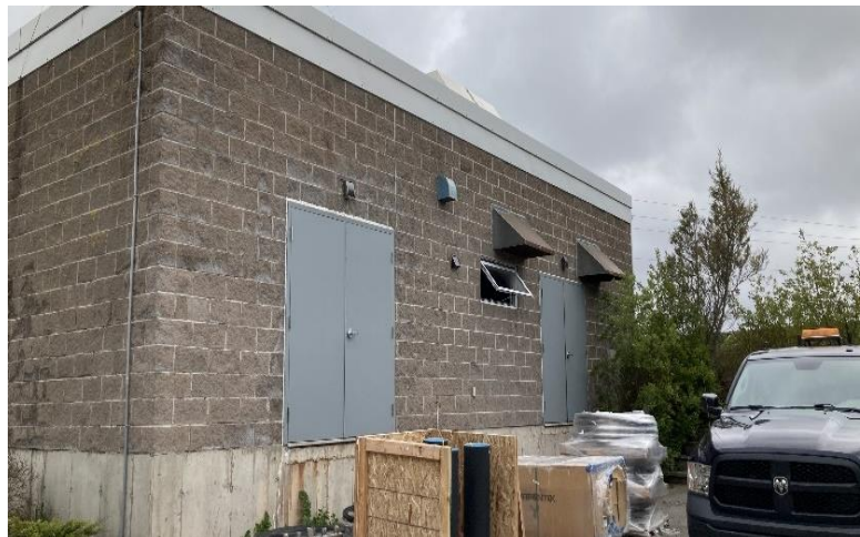
Figure 7.1: Antigonish Wastewater Plant
