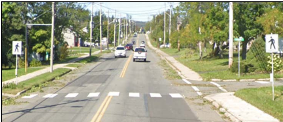
Photo 1 - Example Installation of Crosswalk with RA-4 Signs - Hawthorne Street at Thompson Street
