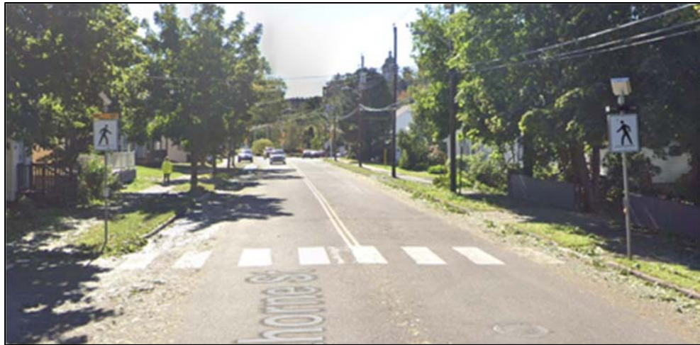
Photo 2 - Example Installation of RRFB - Hawthorne Street at Pleasant Street
