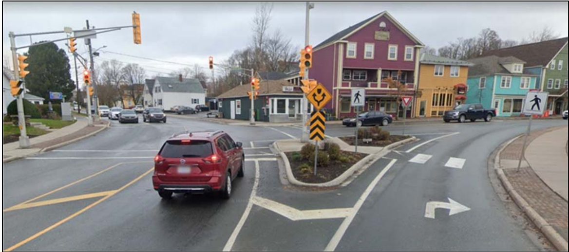
Photo 4 - Example of Markings at a Signal - Main Street at Hawthorne Street
