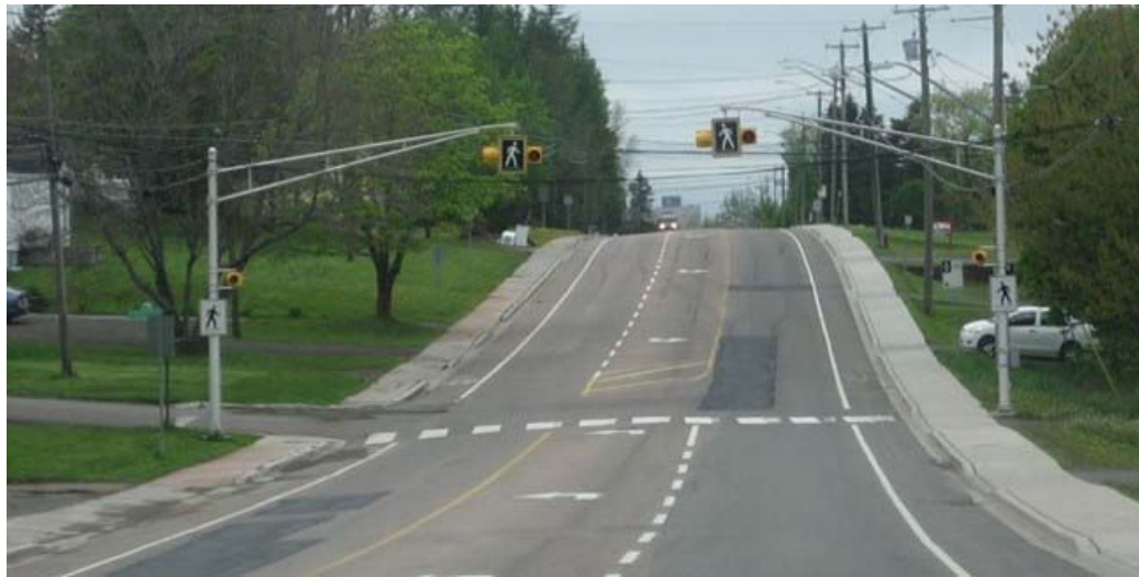
Photo 3 - Example Installation of RA-5 Crosswalk with Overhead Flashing Beacons - Riverview, NB
