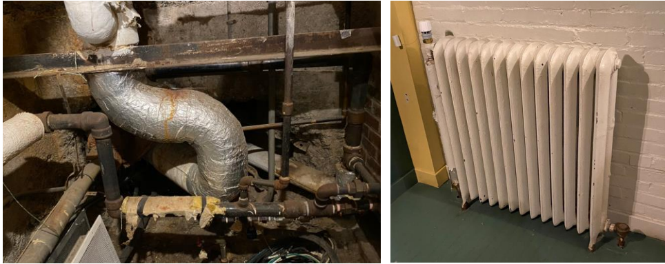
Figure 18: Main steam entrance & cast-iron steam radiator - Bauer theatre
